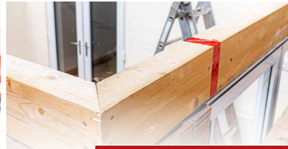
150MM GLULAM EAVES BEAM CUT TO SIZE
