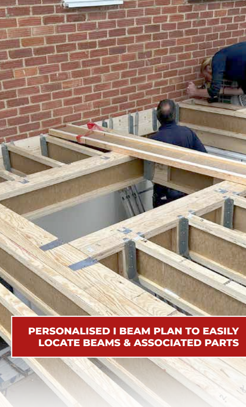
ENGINEERED WALL PLATE WITH GROOVES TO EASILY LOCATE HANGERS
